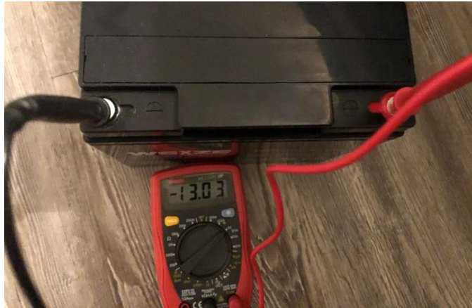
Figure 68: Voltage Testing of the Battery
