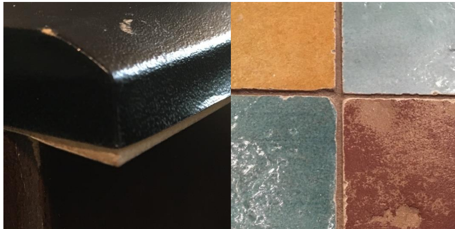
Figure 29- an example of water damaged wood. Figure 29.b- a tiled surface with food trapping grout. Created by Mikey Garrity.
