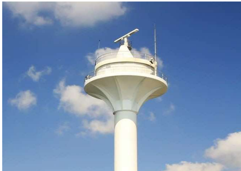
Figure 3.1.2 Unmanned Control Tower
