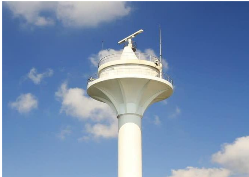
Figure 3.1.2 Unmanned Control Tower
