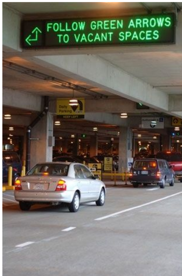
Figure 4.1 - Display at Baltimore/Washington International Airport
