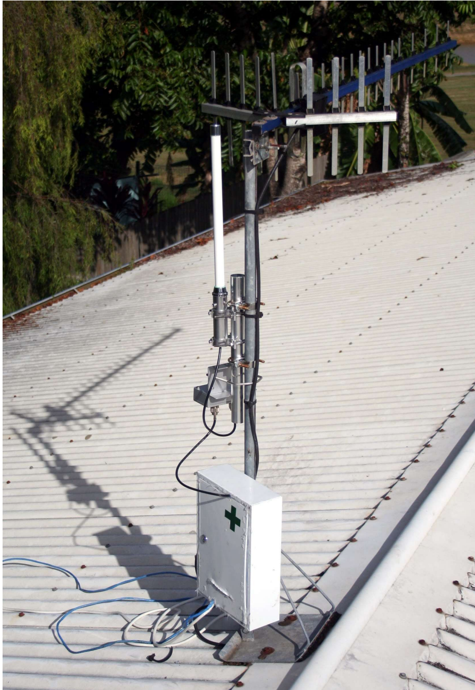
Figure 5.9: Long Range Wi-Fi Amplifier Example (used as part of the public domain)
