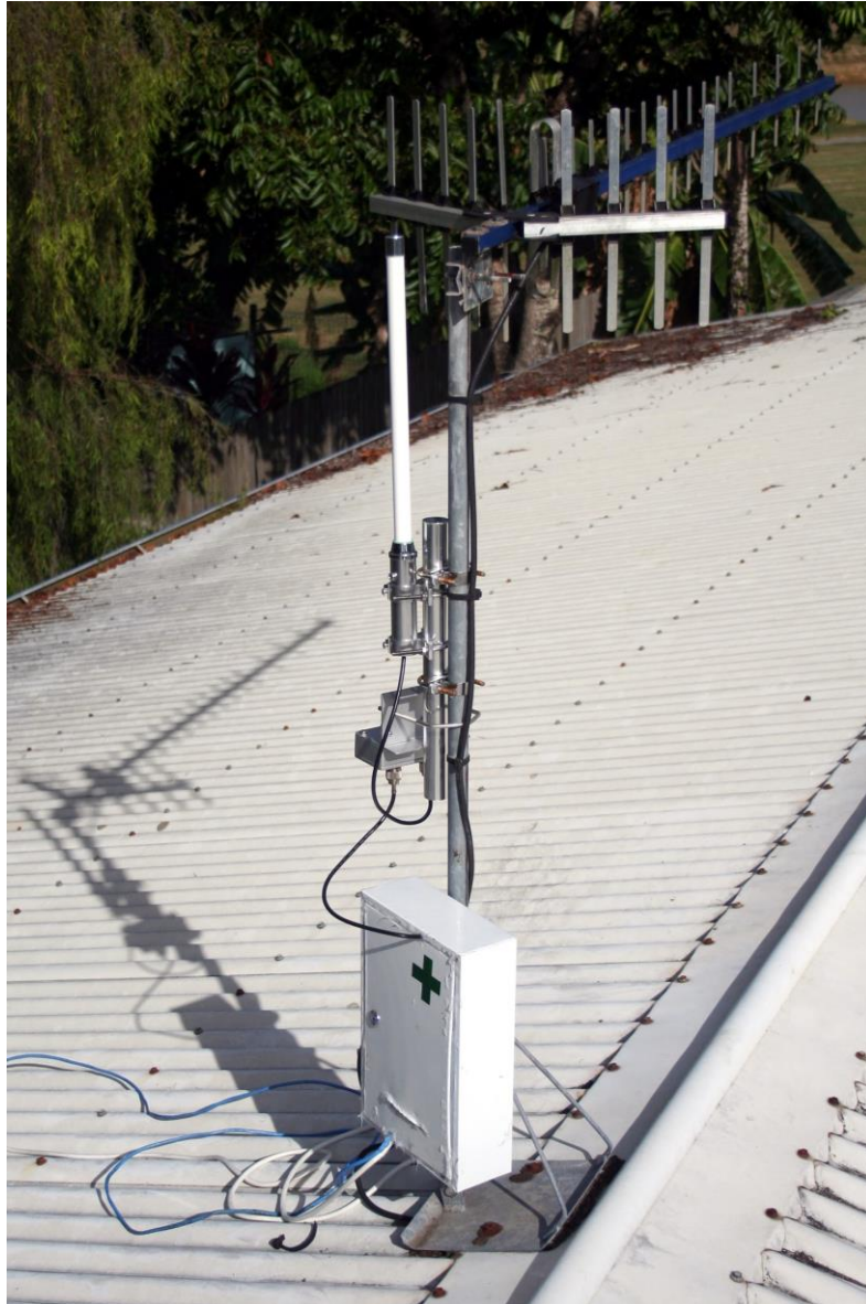
Figure 5.5: Long Range Wi-Fi Amplifier Example (used as part of the public domain)
