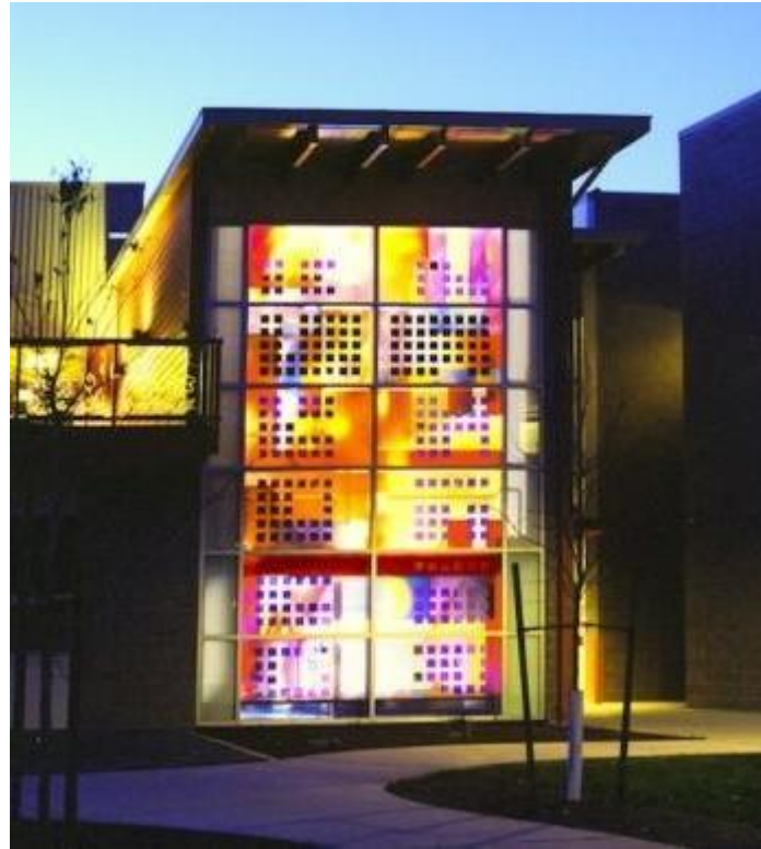
Figure 4.1.3 – PV Stained Glass by Sarah Hall [4.1.2]
